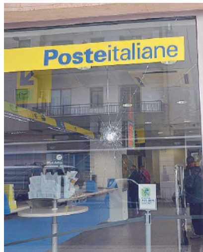
POSTE Disagi in vista
